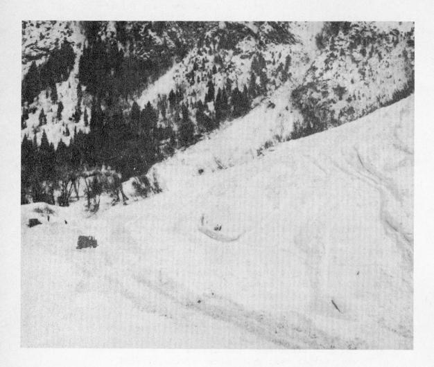
Terminus of the Coal Pit slide showing the characteristic channeling of a wet avalanche. Highway buried 23 feet deep is being uncovered by tractor.
