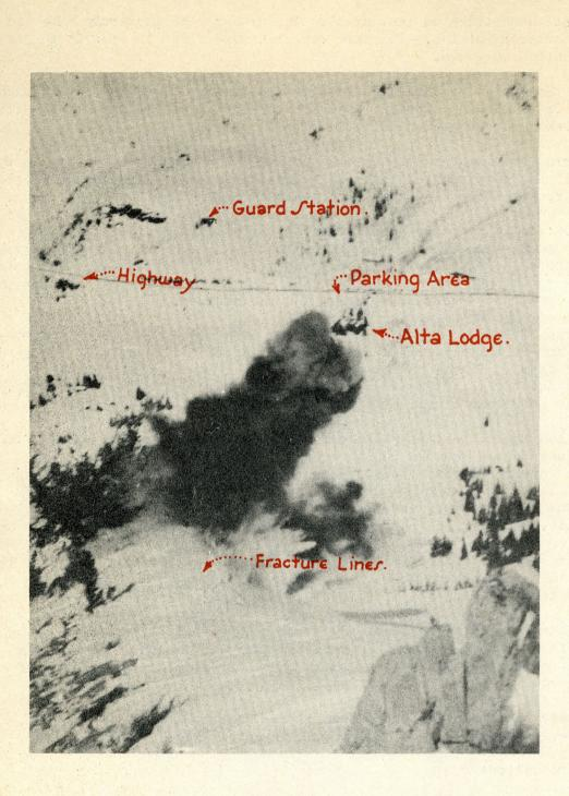
Controlled avalanche blast on Rustler Face. Note the cracks already appearing in the slabbed surface.
