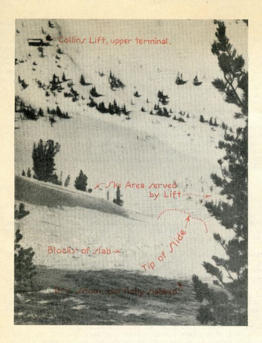
Slab and dry snow avalanche released by explosives and in motion on West Rustler. The tip of the slide is entering the liftserved ski area.
