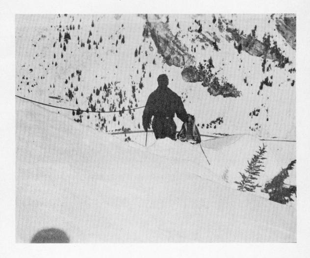
Starting out to plant the explosive charge for cornice removal. Note safety rope.
