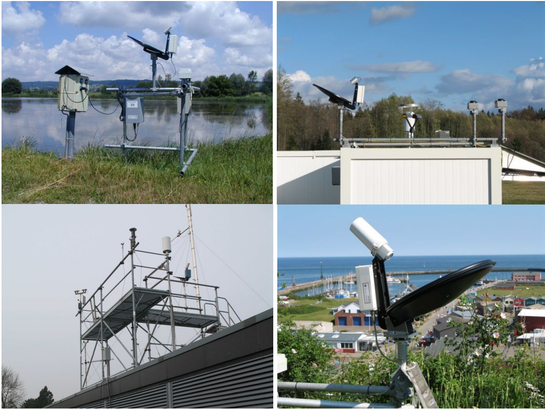
Figure 7 Examples of MRR installations
